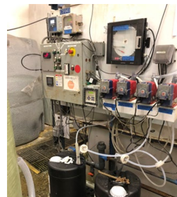
Figure 2: Inspecting Pretreatment System
