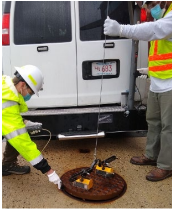
Figure 1: Safely Monitoring Atmosphere
